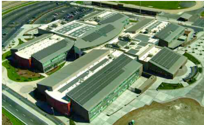
460 kW grid-tied building integrated PV system on Inderkum High School in Sacramento. This is an example of integrating PV in the design process of a new school.
